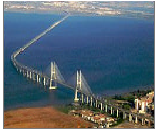
Vasco da Gama bridge, Portugal
